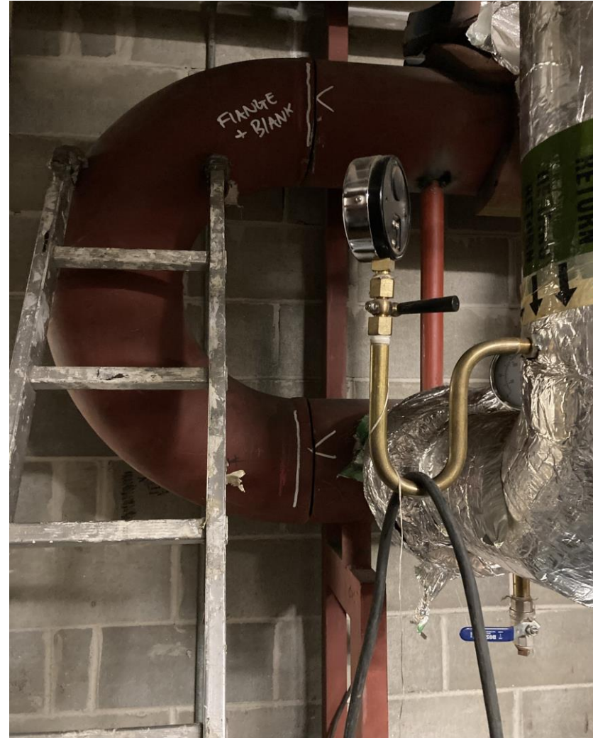
Unnecessary substation, and oversized pipework/low loss header
