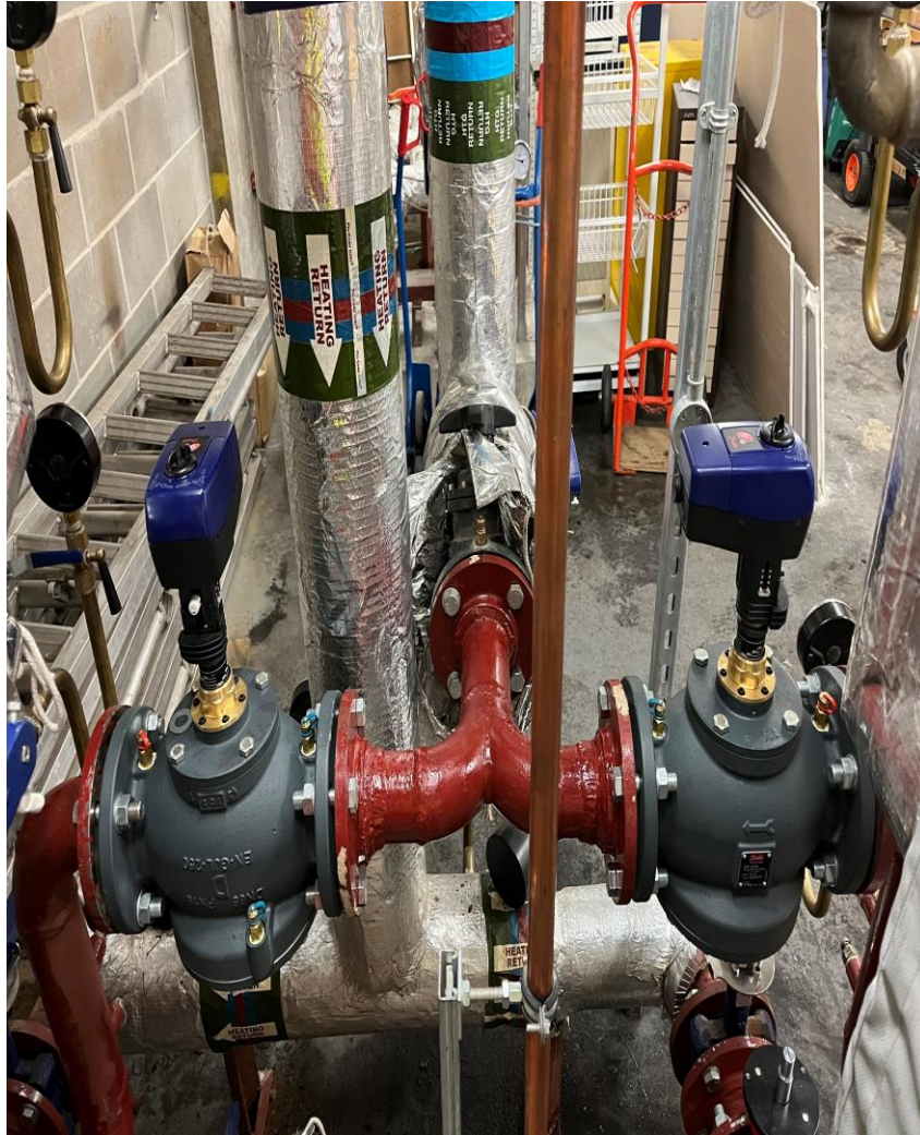
Unnecessary substation, and oversized pipework/low loss header
