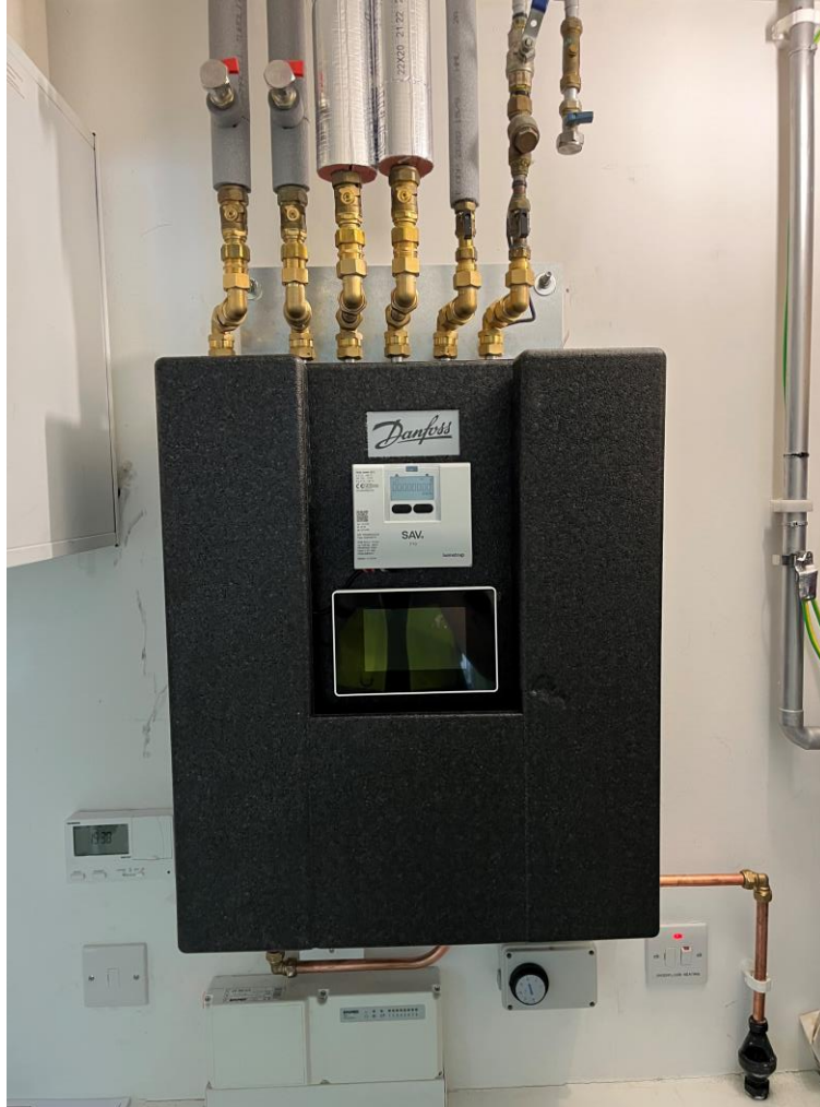
High Performing/Non bypassing Heat Interface Units
